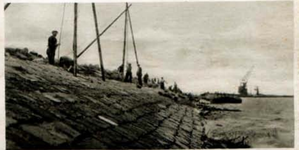
De steenbekleding voltooid
