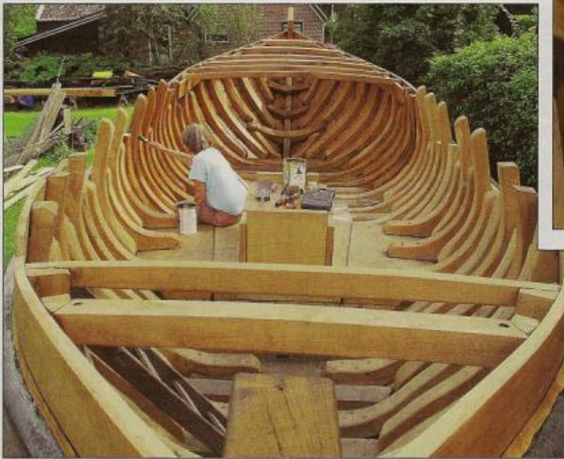
Left —Once the 80 futtocks were replaced, the interior was oiled with a traditional combination of linseed oil and resin called harpuis . Above —Natural crooks were used to make very heavy hanging knees in way of the mast partners. These obviate the need for shrouds, leaving the skuitje’s gunwales clear for handling fishing gear. The box-like structure is part of the livewell, used to keep the catch fresh.
